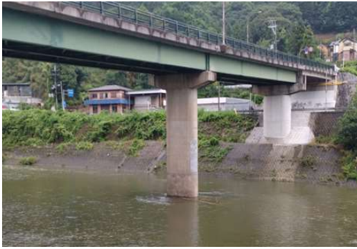
P2橋脚施工前
